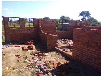
Building in progress
